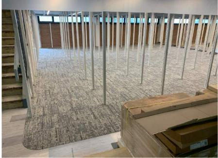
Installed flooring throughout basement and 1st Floor (protected) and support columns under mezz painted
