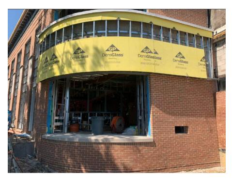
Masonry, roofing, and cornice installed on new addition
