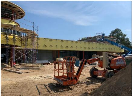
Rotunda and North soffit sheathed with densglas
